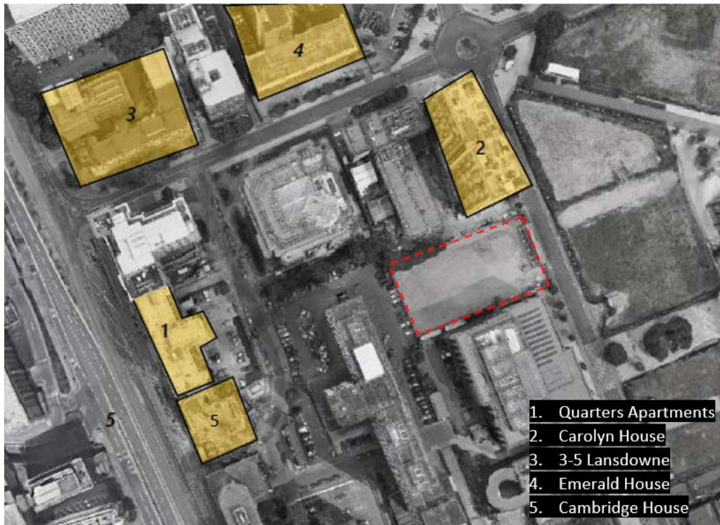
Image 15 – Adjacent residential buildings
